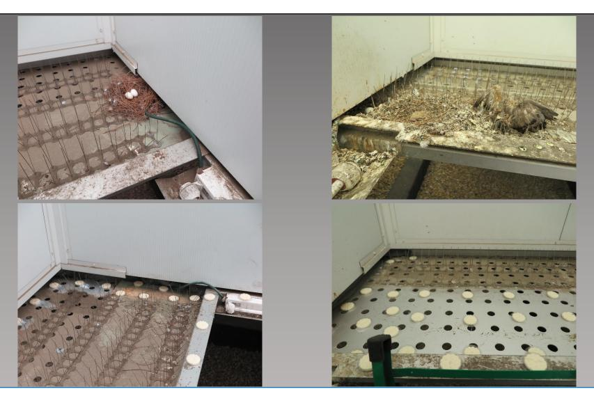
Wherever nests were removed from the flat surfaces at the ends of the skylights, the nesting sites were disinfected (after removing spikes) and treated with dishes of 小島 Bird Free at 15cm centres to prevent further nesting. Dishes were fixed at 20cm centres close to the nesting sites.
