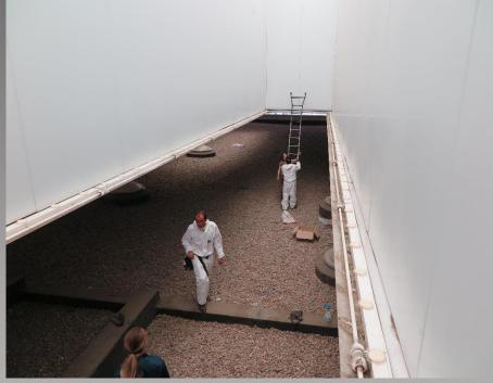
Treatment of skylights 3, 5 6, 8 and 9 was done from ladders. The ledges above the lights on each side of the skylights were cleaned of faeces and treated with dishes of 小島  $Bird\ Free$  at 25cm centres to prevent pigeons from roosting.
